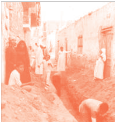
Laying of sewer pipes in Aswan-Nasriya, Egypt /24/
