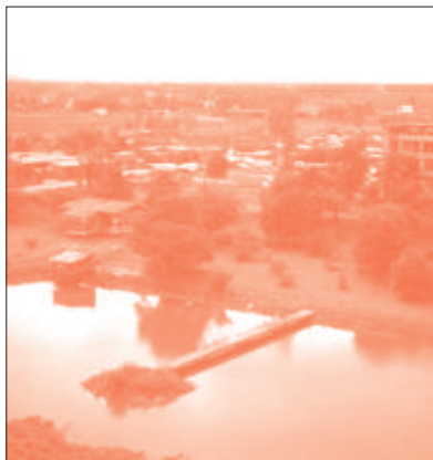
Rainwater retention basin in Phnom Penh, Cambodia /13/
