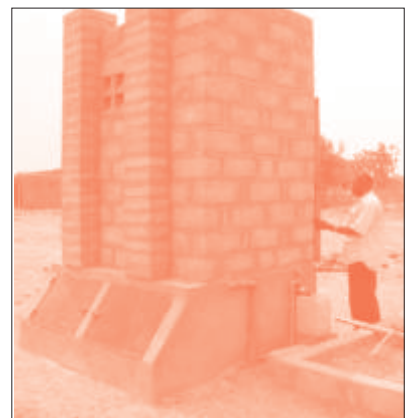
Dry latrine with duplex chamber and separation of urine, Mali
