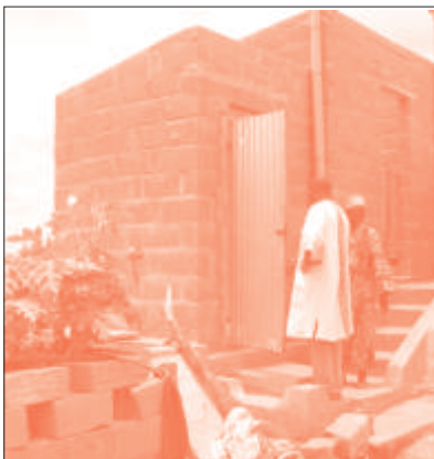
ECOSAN-latrine and grey water irrigation Mali /12/
