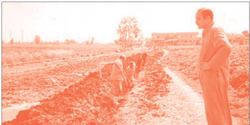
Digging a sewerage trench /25/
