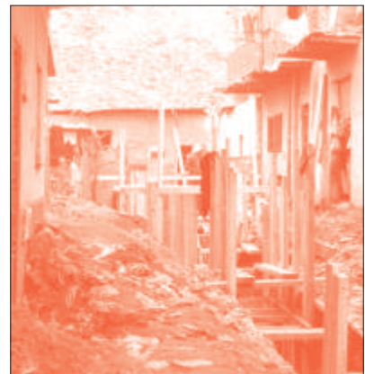
Construction of a sewage system in Cairo, Egypt
