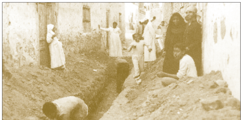
Residents' self-help in installing wastewater pipes in the Urban Upgrading Project Nasriya/Aswan in Egypt
