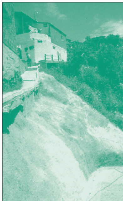
Slope stabilisation in Medellín, Columbia /126/
