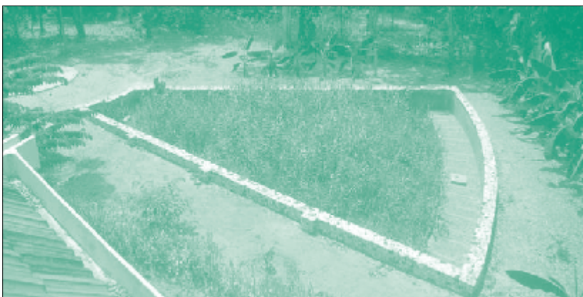
Biological treatment plant in Grace, Auroville, Tamil Nadu, India: Filter basin /110/
