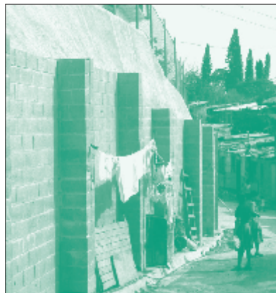
Retaining walls erected in the context of a slum upgrading project /124/
