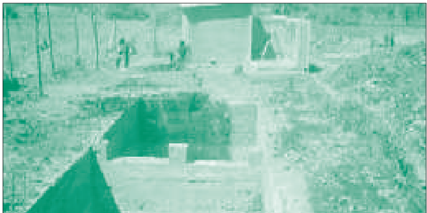
Construction of a septic tank
