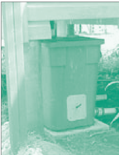
Compost toilet with plastic storage tank /88/
