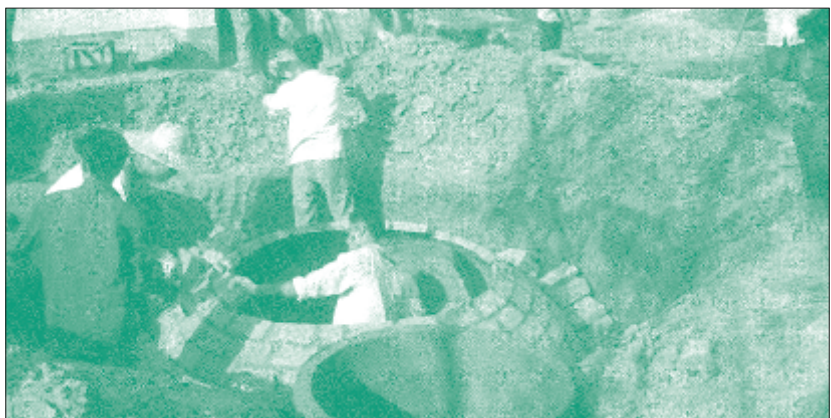
Construction of a Chinese type of biogas plant
