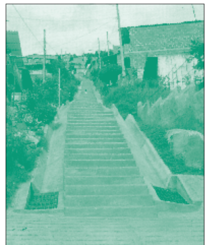
An over-sized drainage canal during the dry season
