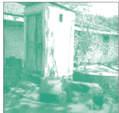
Toilet connected to a Chinese type biogas plant /96/
