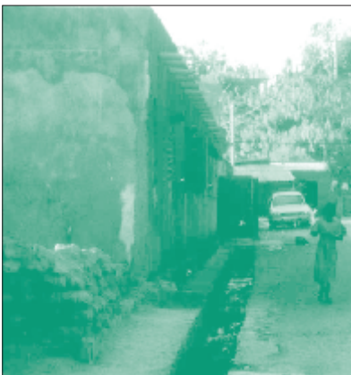
Simple rainwater culvert in Mali
