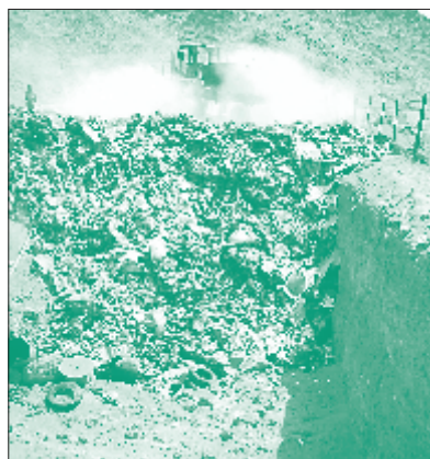
Simple trench landfill in Aqaba, Jordan /66/
