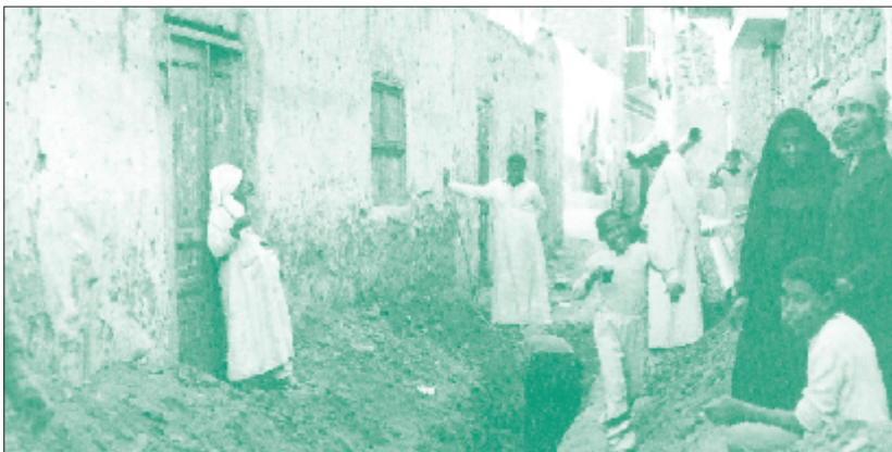
Self-help laying sewage pipes in Aswan, Egypt
