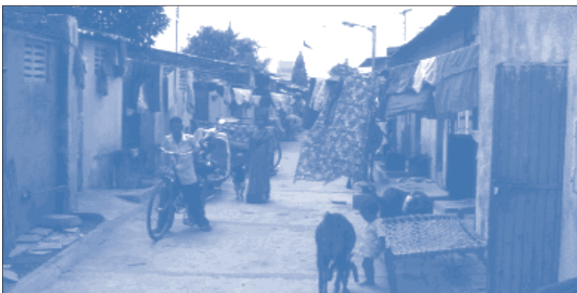
Street after rehabilitation with problematic, semi-open drainage duct in Hanuman Nagar /13/
