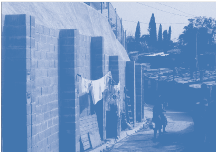
Newly constructed retaining wall to prevent landslides /21/
