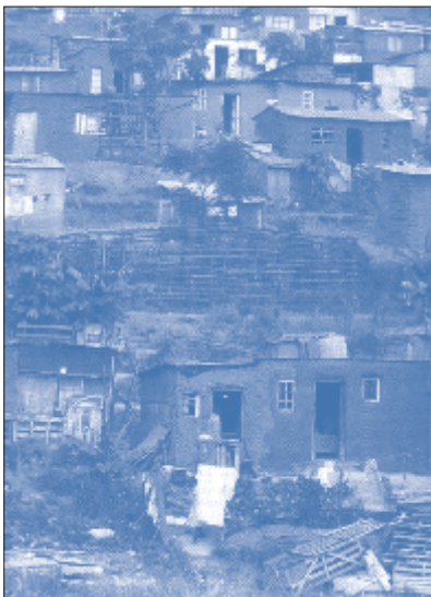
Housing conditions without adequate waste management /4/
