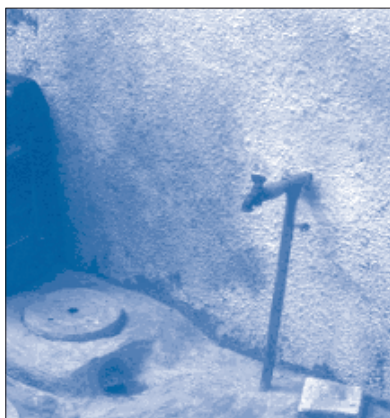
Water connection in Hanuman Nagar /14/
